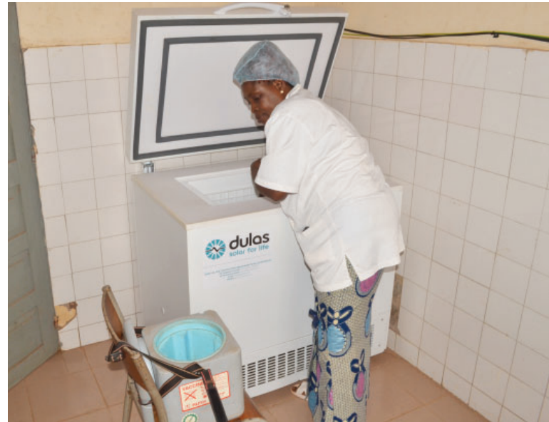
A healthcare professional in Togo using the Dulas VC50SDD solar refrigerator for vaccine storage.
